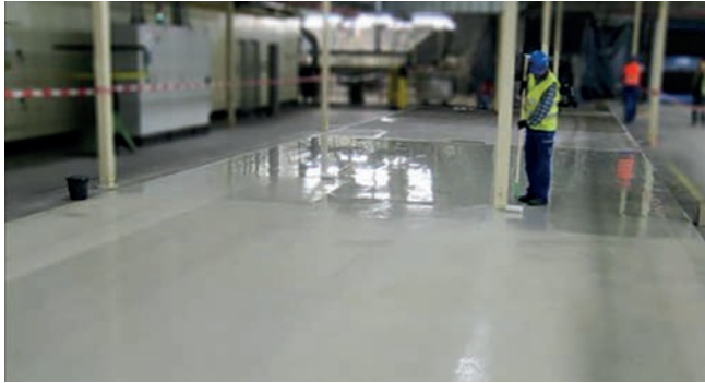
ESKANOL EF floor coating with skid-proof top coating
