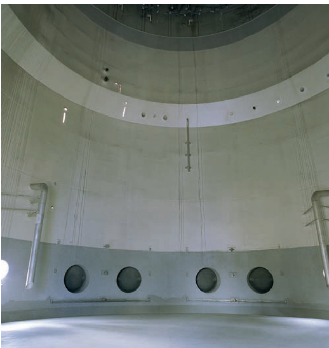
Absorber lined with COROFLAKE 24 and LINING 65 W
