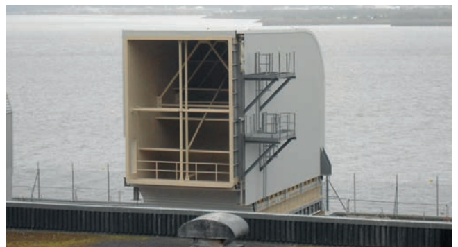
Clean Gas Duct lined with COROFLAKE 24
