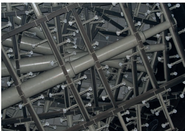
Spray level made of Polypropylen (PP)
