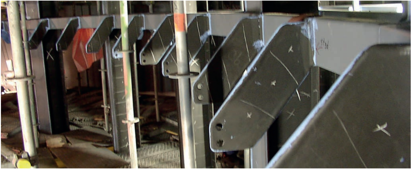
Rubber lined supports in an absorber
