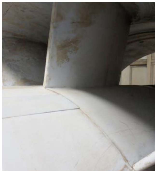
REMAFLON (PTFE) as nonstick lining in a flue gas fan
