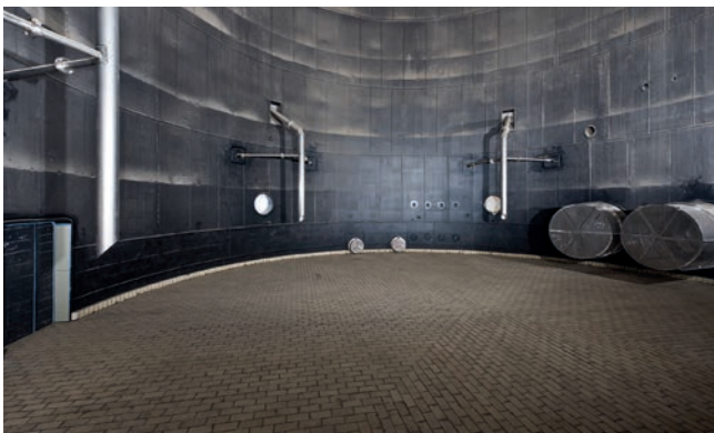
Floor of an absorber rubber lined with CHEMOLINE 4 B and additional brick lining with CHEMOKITT FU 1310
