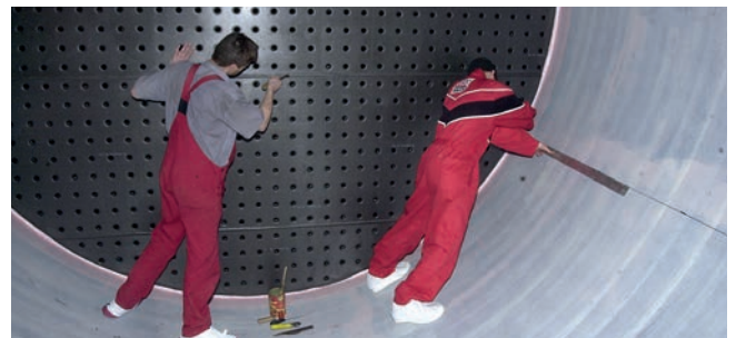
Lining of a filter tank
