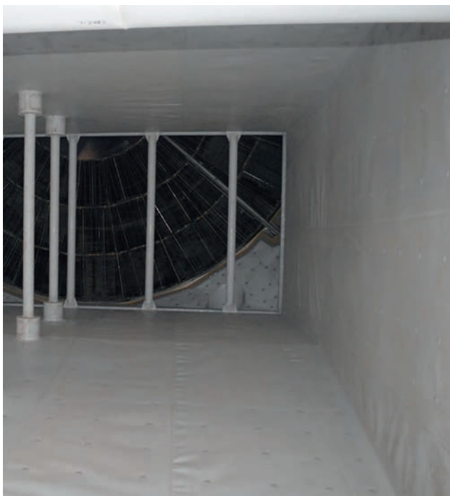
PTFE-M lining in a raw gas duct
