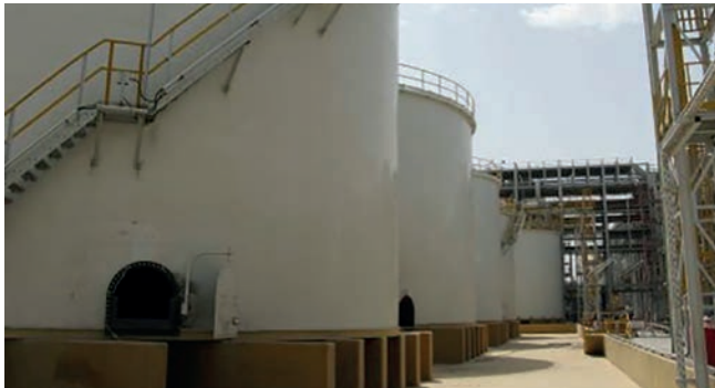
Coated secondary containment
